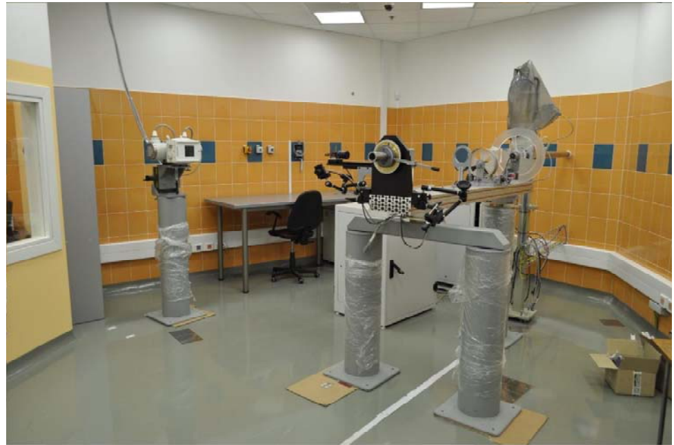
Installation of the new eye line at NCRH-CCB
