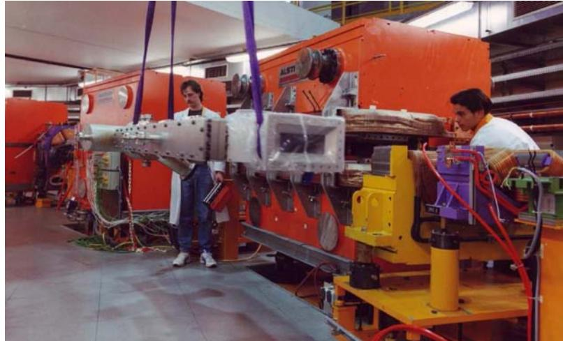
**Figure 2.3:** The special COSY-11 vacuum chamber during installation.
