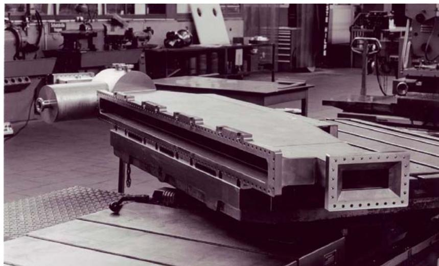
**Figure 2.5:** The COSY-11 vacuum chamber during construction at the ZAT of the Research Center Jülich.
